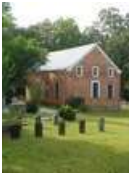
Old Brick Church, Little River, SC
